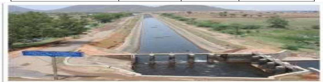
(A): Start Point of Canal
